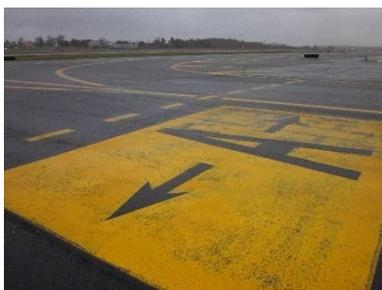
Surface painted taxiway direction signs have a yellow background with a black inscription, and are provided when it is not possible to provide taxiway direction signs at intersections, or when necessary to supplement such signs. These markings are located adjacent to the centerline.
