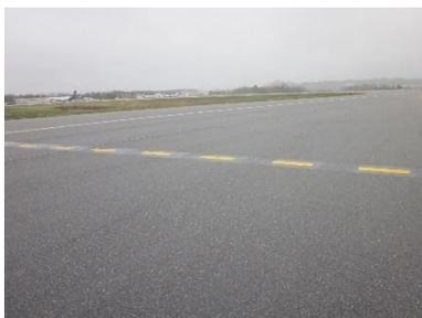
A taxiway intermediate holding position marking is painted as a broken yellow line across a taxiway that is perpendicular to the taxiway centerline. At the Jetport taxiway intermediate holding position markings are located at the intersection of Taxiways A and C. They are used to advise a pilot or driver where to hold short on a taxiway, when instructed by the air traffic control tower to "hold short of either: Taxiway A (when on Taxiway C), or Taxiway C (when on Taxiway A).
