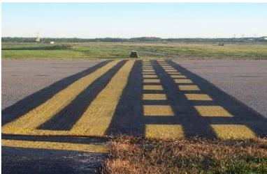
Runway-Holding Position Markings are painted surface markings used to denote the entrance of a runway from a taxiway. These markings also show you where to “hold-short” for a runway when instructed to do so.
