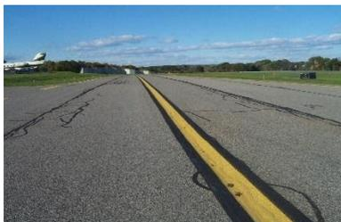
Taxiway centerline markings are a single solid line down the middle of a taxiway that inform a pilot or a vehicle operator of where the middle of the taxiway is. Most aircraft are taxied (driven) down the middle of the taxiway to ensure that they have the most wingtip clearance available on either side.
