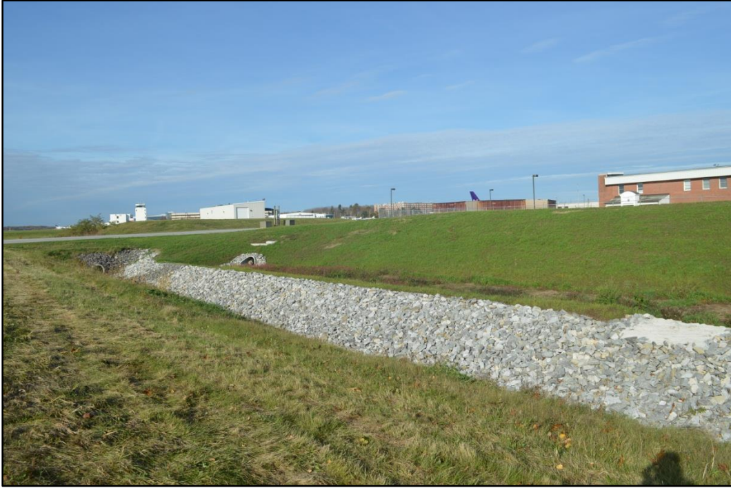
Plate 1. Drainage features in SA-2, view northwest.
