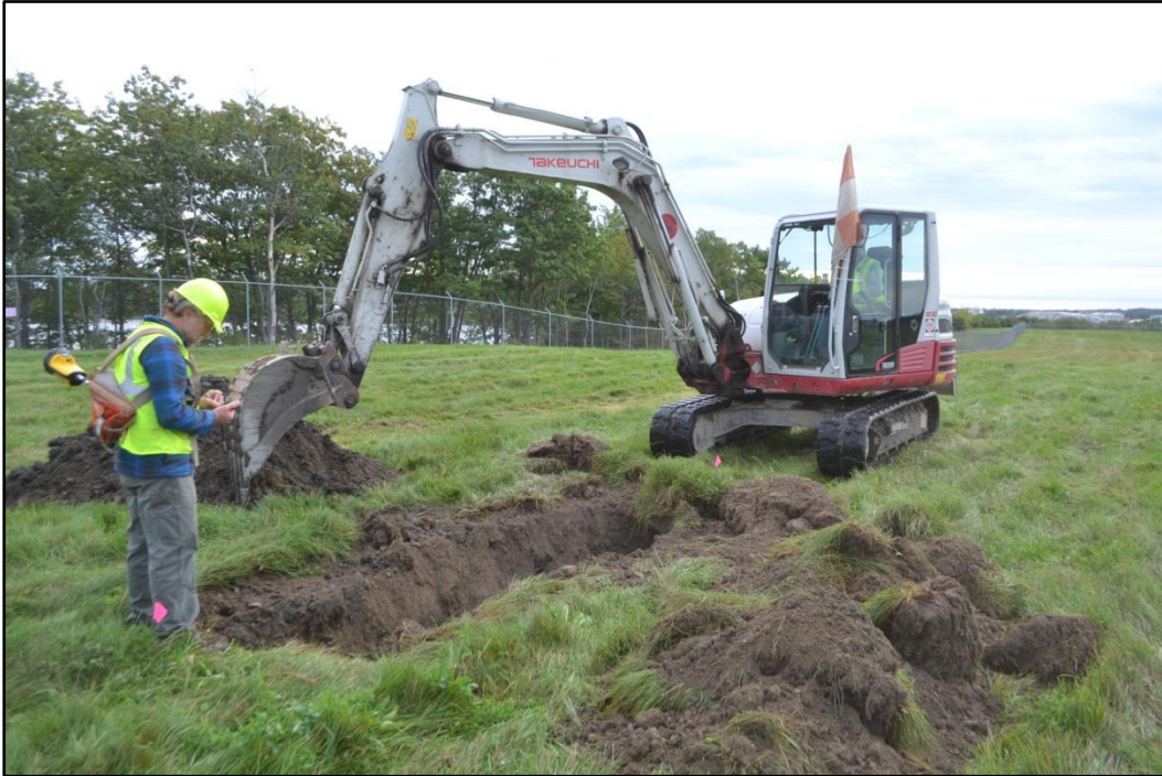
Plate 12. Trenching in progress in water quality filter area, view south-southeast.
