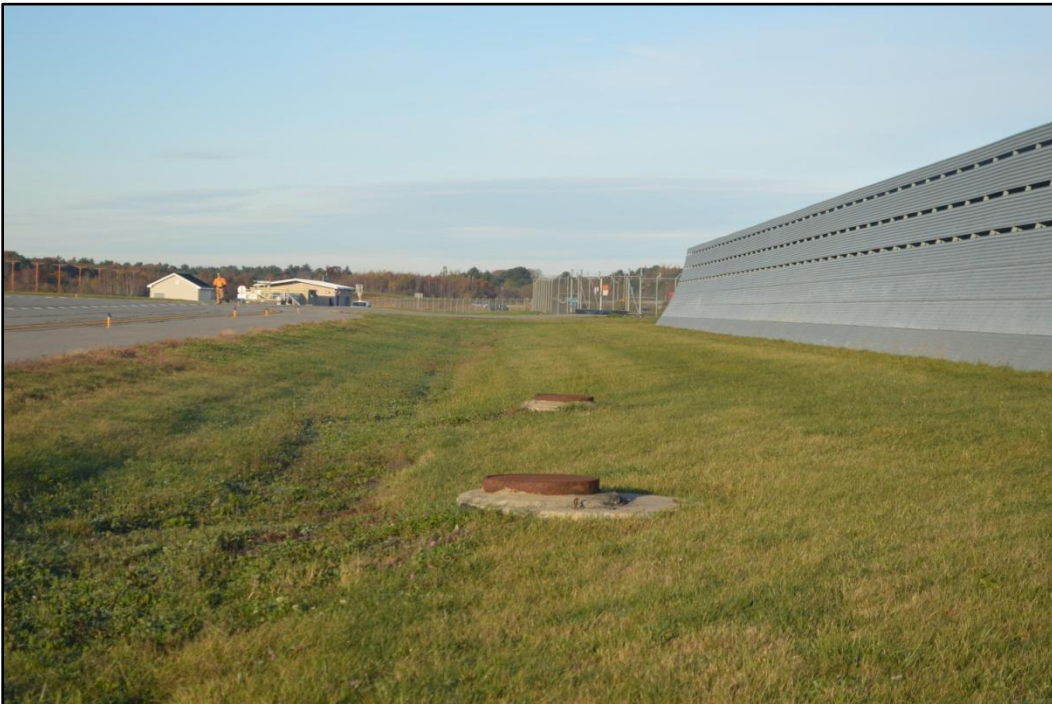
Plate 6. Buried utilities and sound wall in MU-1, view west.
