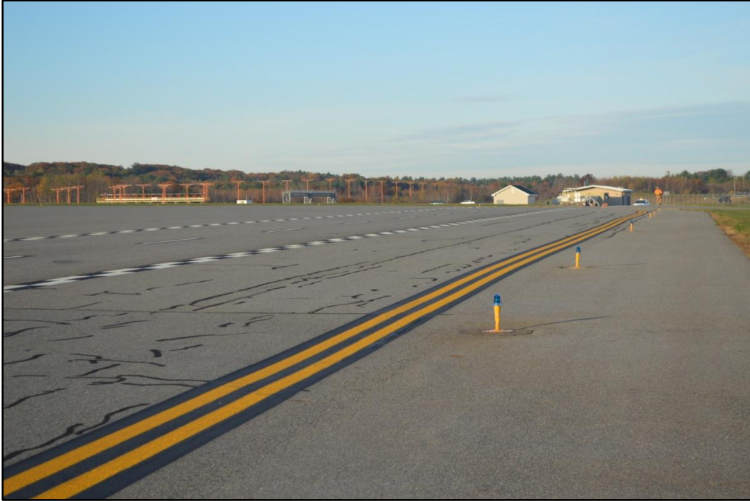
Plate 7. Section of extant taxiway and lighting system that dominates MU-1, view southwest.
