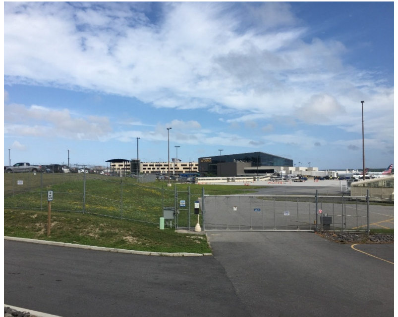
Figure 5: Pole-mounted parking lot and apron lights west of the terminal building
