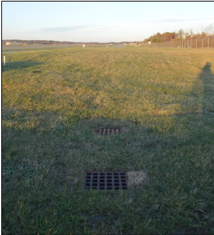
Plate 9. Drainage features in MU-2, view west.
