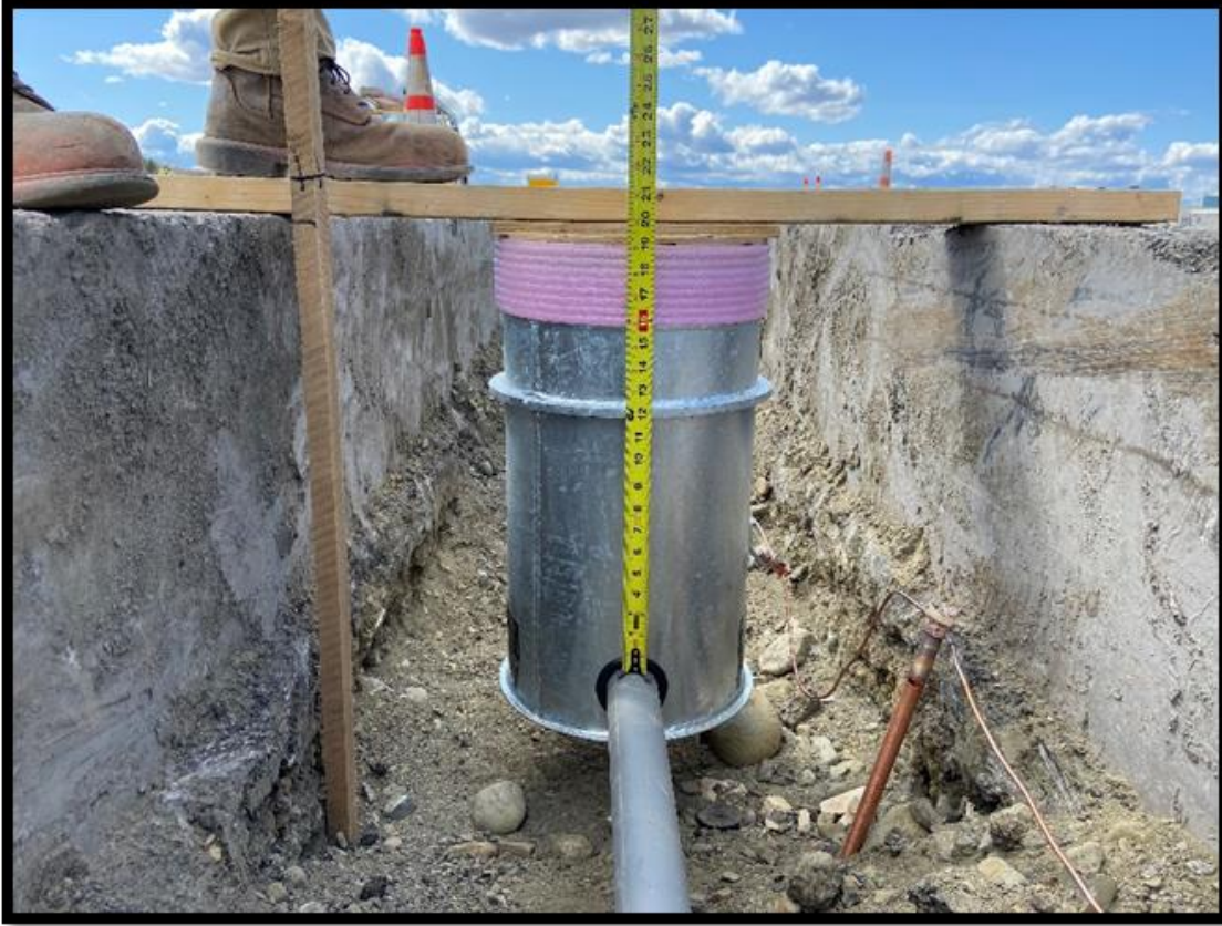
Runway Centerline Light Installation
