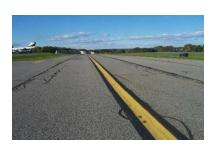
Taxiway centerline markings are a single solid line down the middle of a taxiway that inform a pilot or a vehicle operator of where the middle of the taxiway is. Most aircraft are taxied (driven) down the middle of the taxiway to ensure that they have the most wingtip clearance available on either side.
