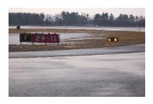
Elevated Runway Guard Lights are located within the vicinity of runway holding position markings and runway holding position signs, where taxiways intersect a runway. These lights provide additional warning to a driver that he or she is about to enter onto a runway. Runway guard lights are yellow in color, and are comprised of two lights that alternate on and off in sequence. These lights are located on both sides of a taxiway when that taxiway intersects a runway.
