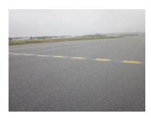
A taxiway intermediate holding position marking is painted as a broken yellow line across a taxiway that is perpendicular to the taxiway centerline. At the Jetport taxiway intermediate holding position markings are located at the intersection of Taxiways A and C. They are used to advise a pilot or driver where to hold short on a taxiway, when instructed by the air traffic control tower to "hold short of either: Taxiway A (when on Taxiway C), or Taxiway C (when on Taxiway A).
