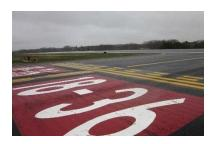
A surface painted holding position sign provides supplemental visual cues that alert pilots and vehicle drivers of an upcoming holding position location and the associated runway designator(s) as another method to minimize the potential for a runway incursion.
