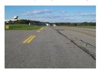
A taxiway edge marking is always painted as a double yellow line. They are used to advise a pilot of where the taxiway edge is located. When a plane is not permitted to turn off from a taxiway, the edge lines will be solid. When a plane is permitted to turn off from a taxiway and onto another paved area, like an Apron for instance, the edge lines will be dashed (broken). In the picture above, the dashed taxiway edge line means that a driver can
