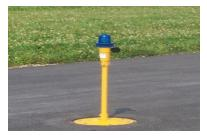
Taxiway edge lights are always blue in color. These lights are used at night and during bad weather conditions to illuminate the taxiway's route and to delineate where the edges are located.
