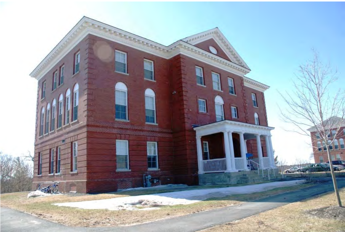
12. Portland International Jetport—Visual Assessment, Portland, ME. View of Cottage #5, State Reform School/Brick Hill Historic District, S. Portland, Photographer facing SW, April 2008
