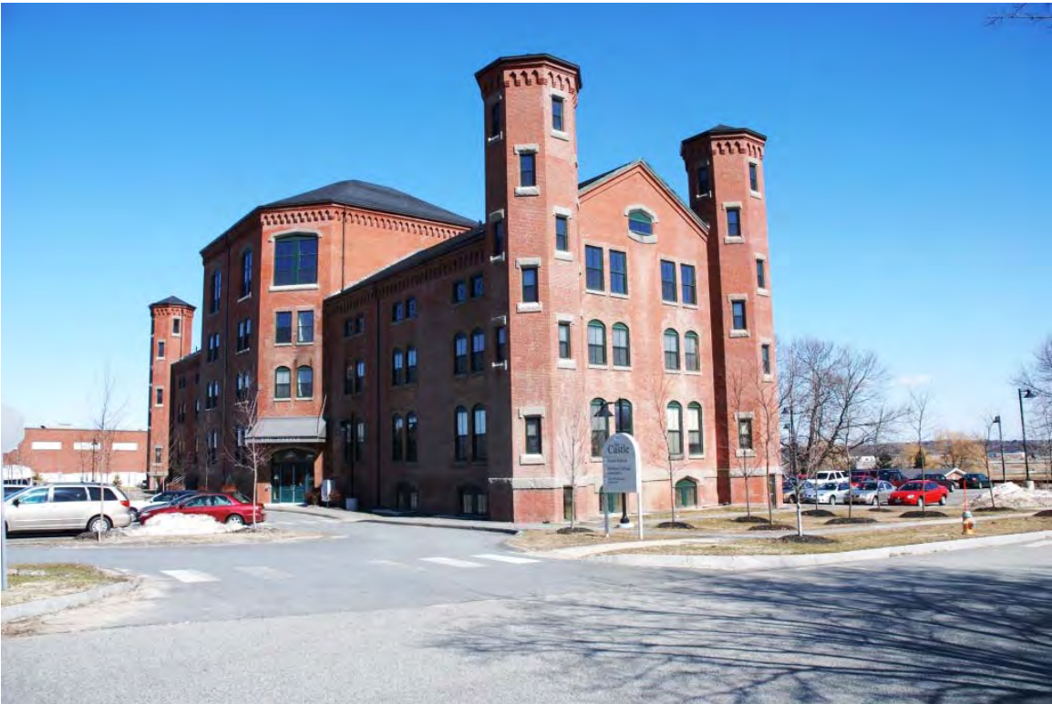
2. Portland International Jetport—Visual Assessment, Portland, ME. View of Administration Bldg., State Reform School/Brick Hill Historic District, S. Portland, Photographer facing NE, April 2008
