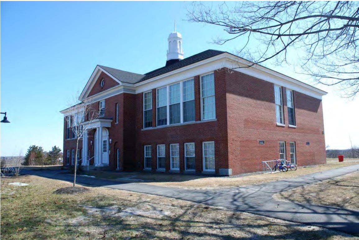
8. Portland International Jetport—Visual Assessment, Portland, ME. View of A.R. Gould School, State Reform School/Brick Hill Historic District, S. Portland, Photographer facing E, April 2008
