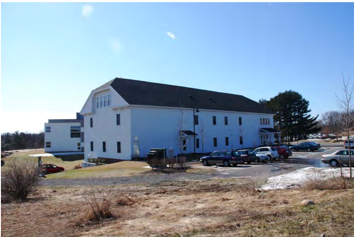
6. Portland International Jetport—Visual Assessment, Portland, ME. View of Grounds Building, State Reform School/Brick Hill Historic District, S. Portland, Photographer facing S, April 2008
