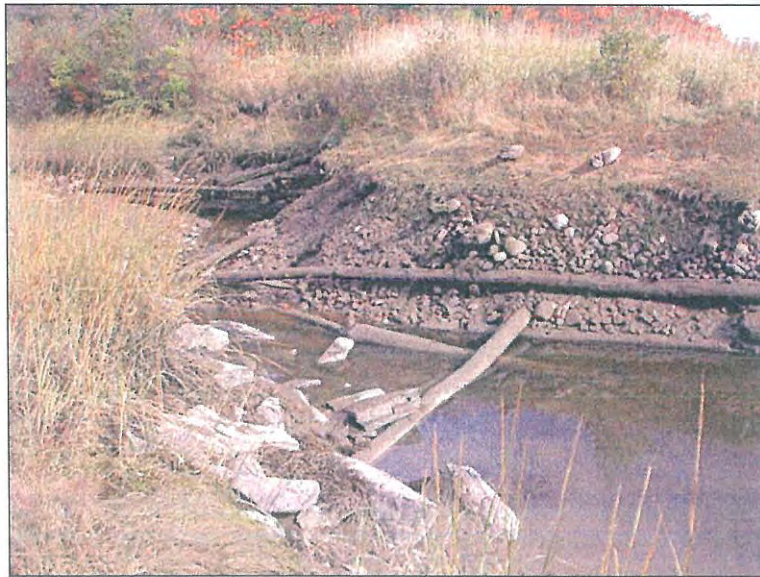
Plate 4. Wharf remains, looking northeast.
