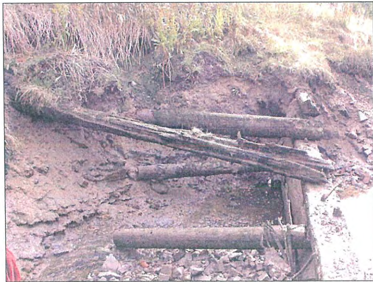
Plate 6. Interior of cribbing, looking east.
