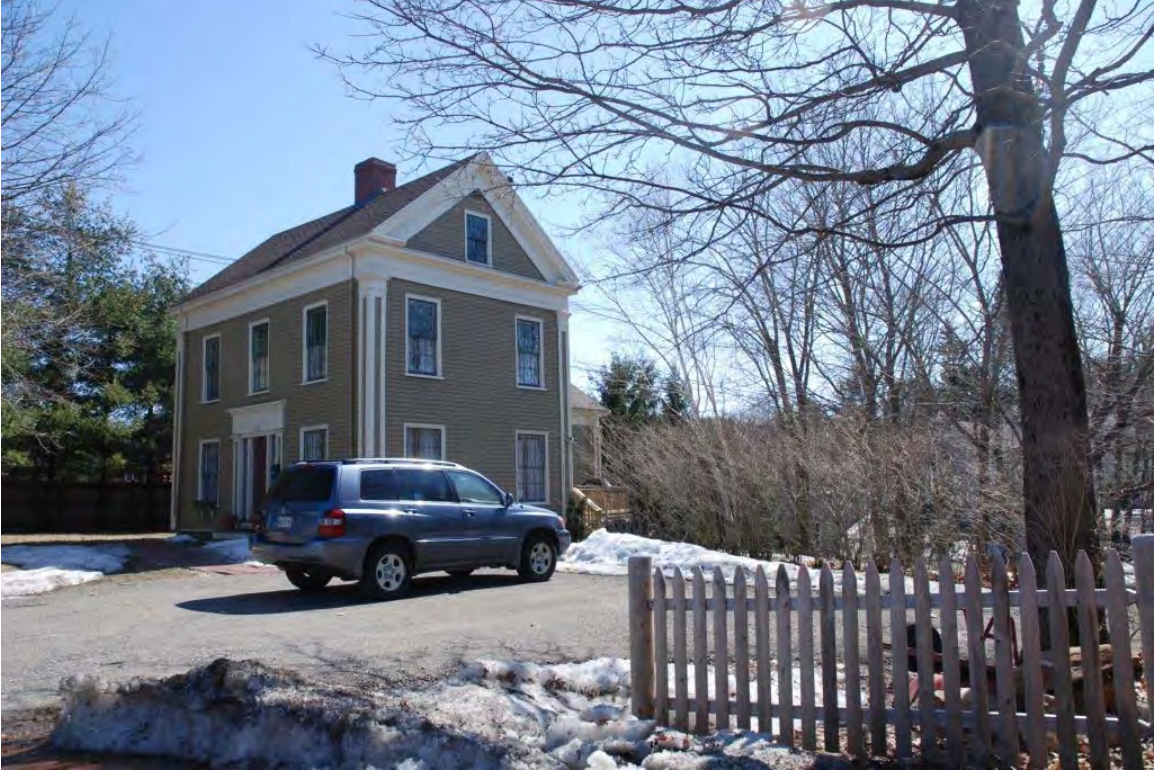
51. Portland International Jetport—Visual Assessment, Portland, ME. View of house at SW corner of Westbrook and Congress Streets, Stroudwater Historic District, Portland, Photographer facing SW, April 2008
