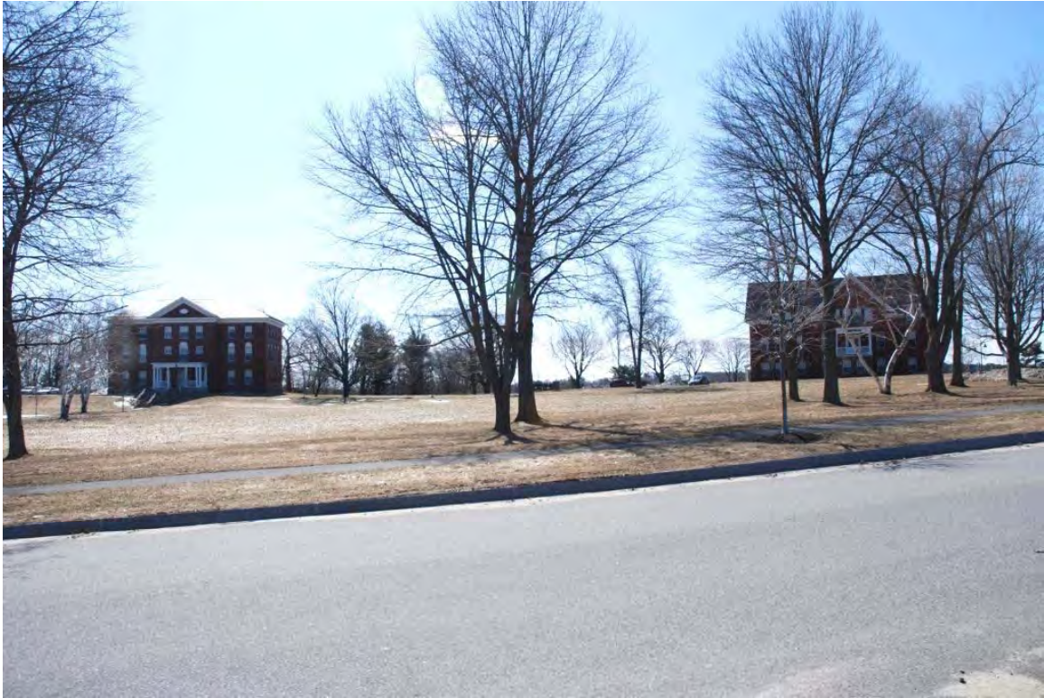
17. Portland International Jetport—Visual Assessment, Portland, ME. View of Cottages #2 and Cottage #3, State Reform School/Brick Hill Historic District, S. Portland, Photographer facing S, April 2008
